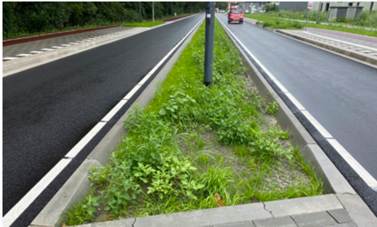
Water infiltratieberm (Bronvermelding: RHDHV)
